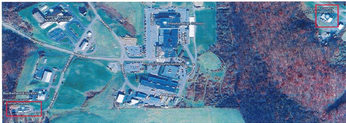
Figure I.A.1.2: Preston County Facilities Aerial View – Animal Shelter and OEM/911
